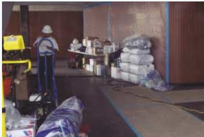
Construction workers repairing the damage caused by the fire and smoke.
